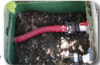
Swing Joint Connection
